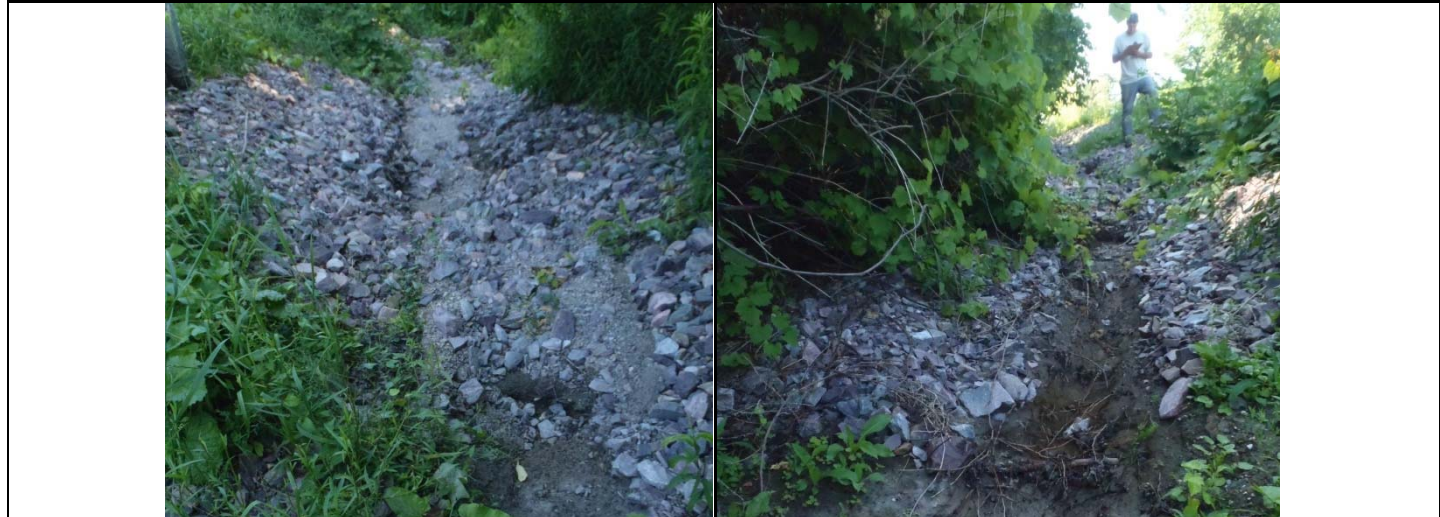
Photo 1. Looking down riprap Photo 2. Looking up riprap, channeling
