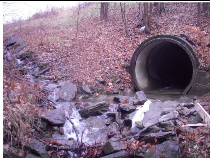
Photo 1. Looking upstream at culvert under I-89 N.Bound
