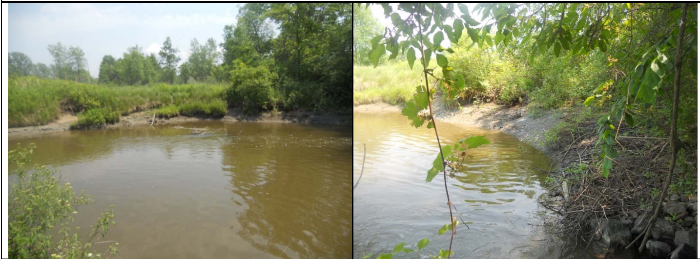
Photo 1. Scour pool at outfall
