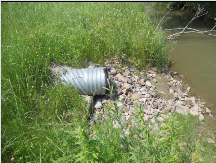
Photo 1. Recent riprap around culvert
