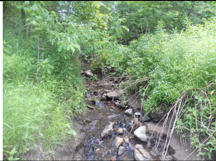
Photo 1. Bank erosion in tributary
