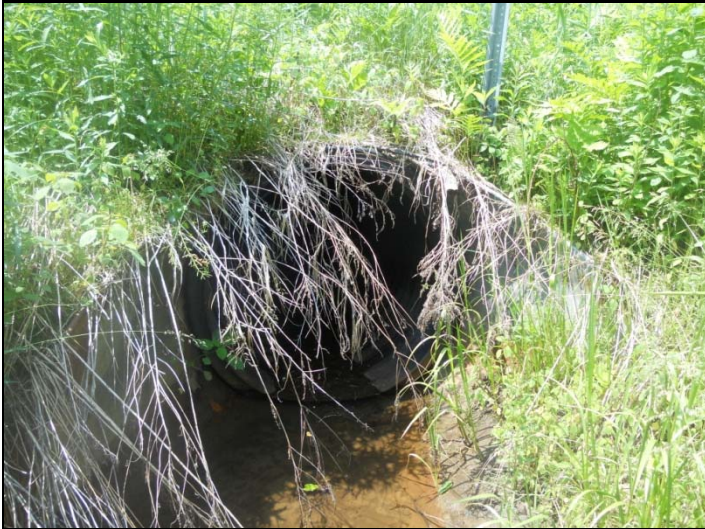
Photo 1. Existing 36" plastic culvert
