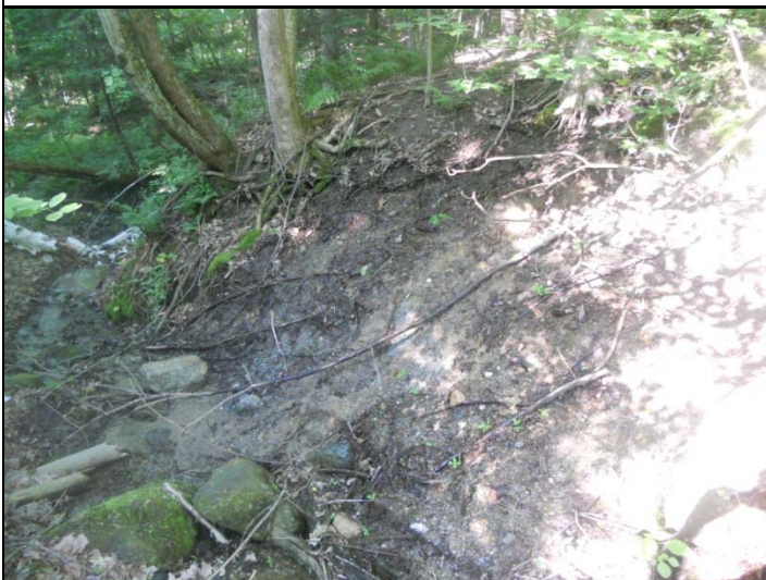
Photo 1. Bank erosion in channel
