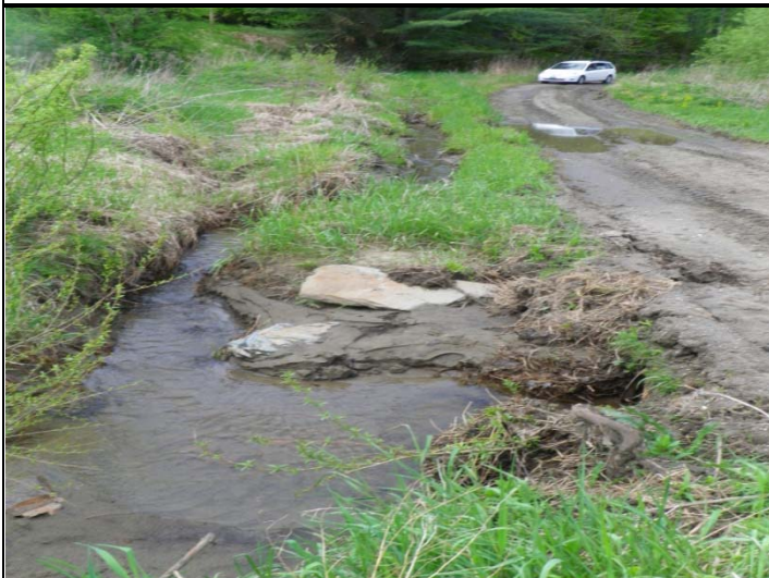
Photo 1. Straightened stream flowing to culvert
