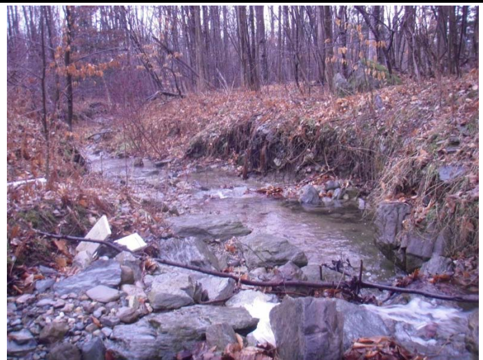
Photo 2. Looking downstream from culvert under I-89.
