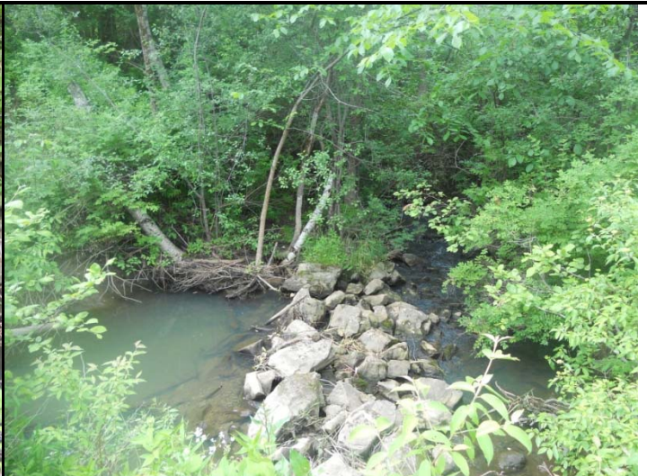
Photo 2. Upstream rock weir causing pooling
